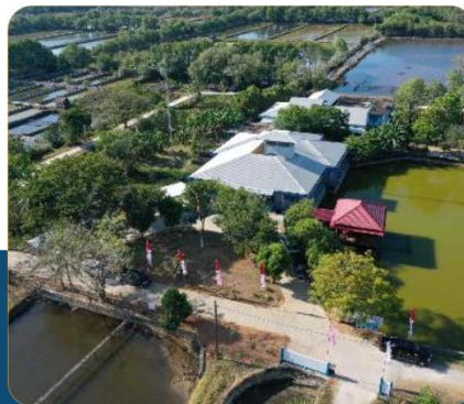
Instalasi Tambak Silvofishery Marana
