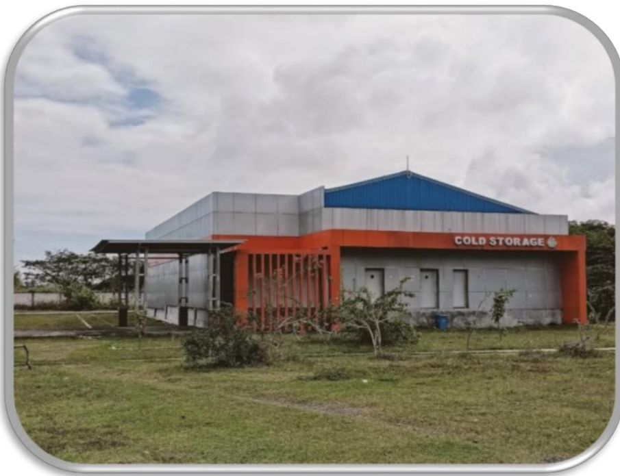
Cold Storage Luas 616 m2
