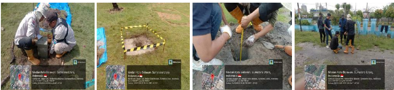
Pemasangan Benchmark (BM) di halaman kantor PPS Belawan & Guest House
