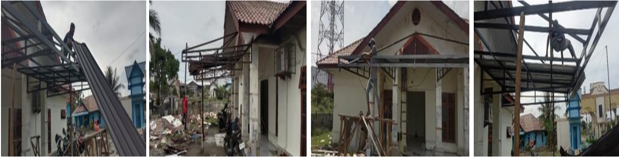
Pemasangan Kanopi Guest House
