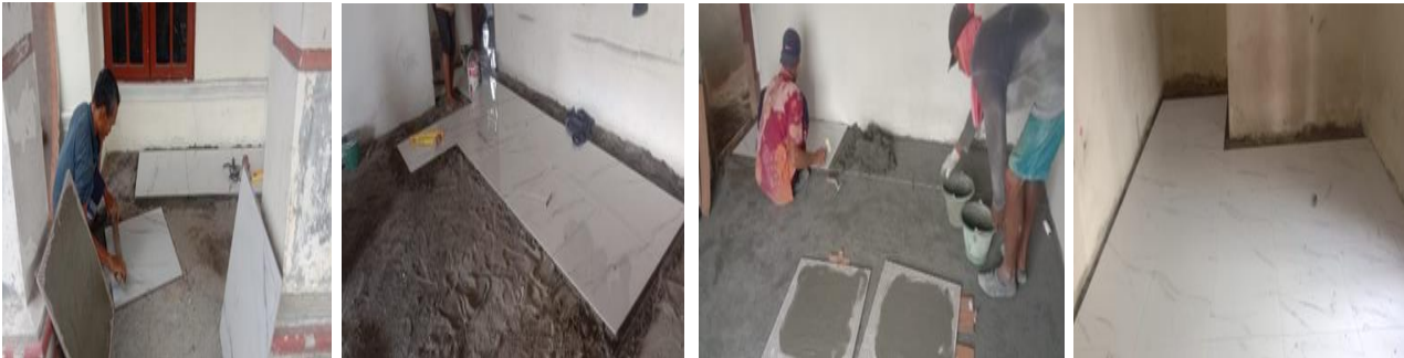
Pemasangan Keramik Guest House
