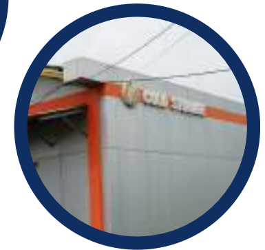
Cold Storage KKP cold storage
