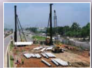
Piles Foundation for Bridges
