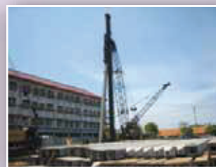
Piles Foundation for Building
