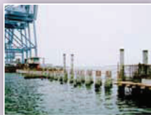
Piles for Marine Structure
