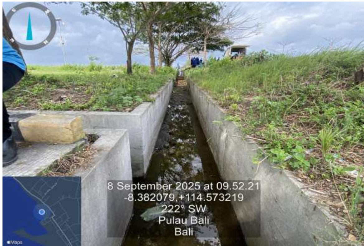
Drainase Ujung Barat Break Water
