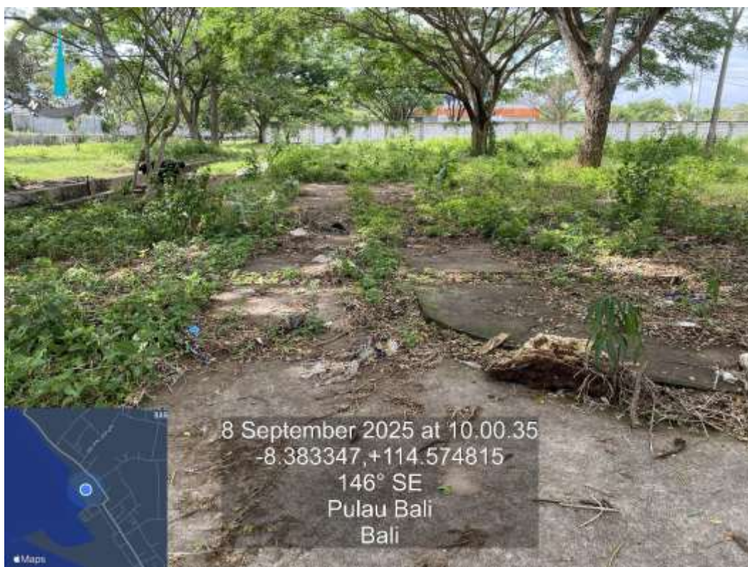
Trotoar Sekeliling Cool Storage Kiri
