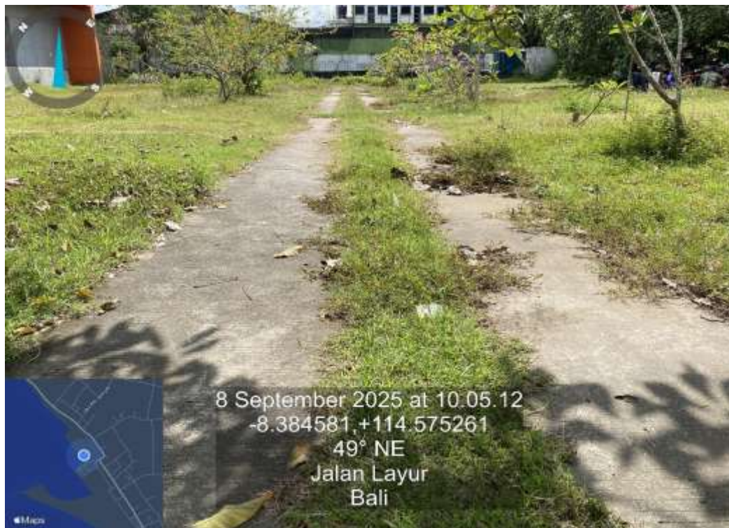
Trottoar Sekeliling Cool Storage Kanan
