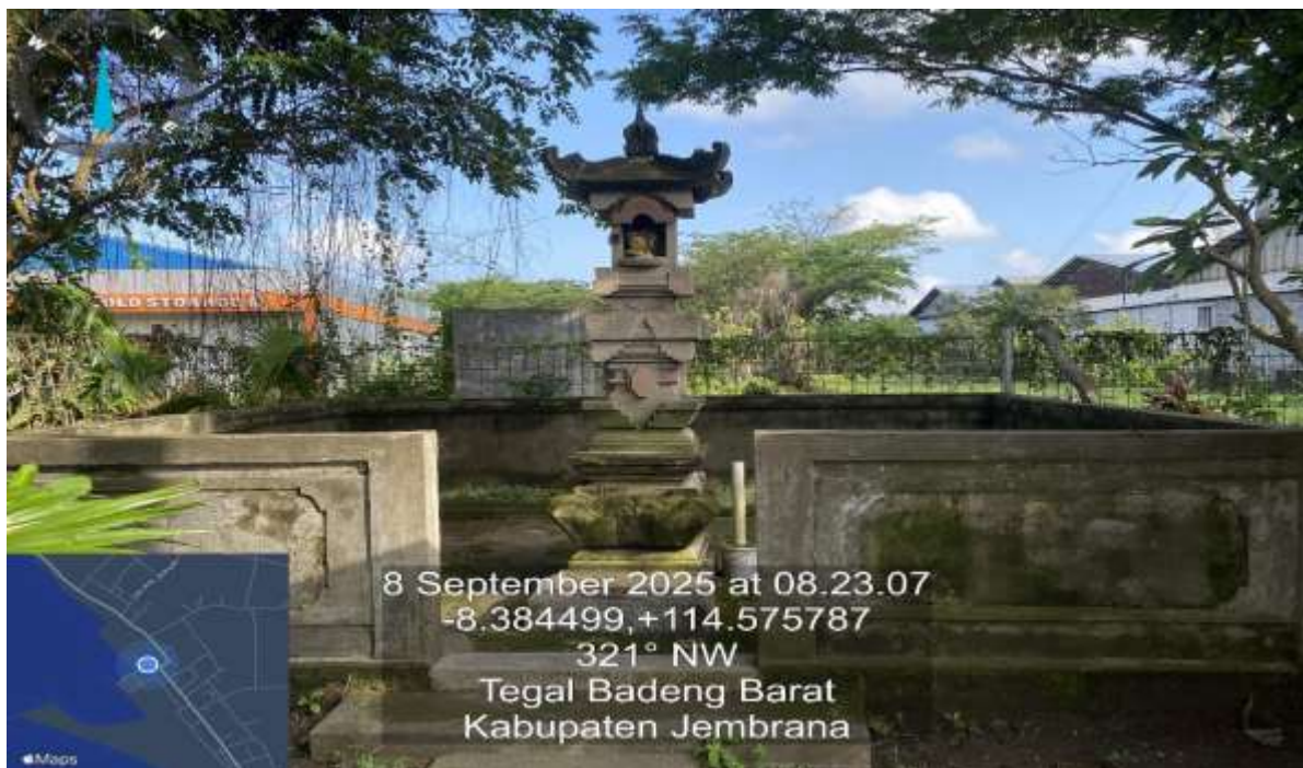
Pura Samping Toilet
